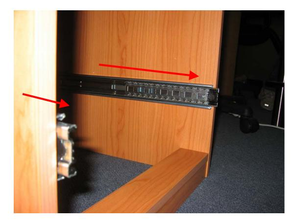
3. Connect the Triple slide rail and roller as shown below
